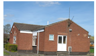
OAP Community Centre, Open Acre, Ironville NG16 5QA
